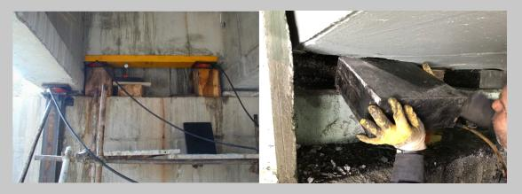
Note the dial gauge reading if required and mark the existing pad position one by one and then remove it and replace the new bearing pad in same position one by one. After successfully replacement, release the pressure of jacks and load is again on the structure. Remove the jacks and again do the same procedure to next side of the span if needed.
