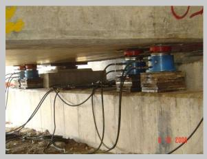
3. For all hydraulic jack one hydraulic pump is enough with the help of manifold lines part. Hydraulic Pump is activated through the three phase generator. After that all the jacks would be fixed by giving some pressure to touch the below surface of girder. Packing of small plates can be used if required to touch the surface. This step can be done to all the jacks one by one to sure that they take the load at once for complete one side span of the bridge.
